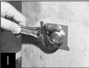
Removing skid from bottom of cabinet.
