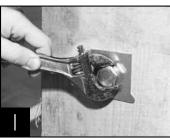
Removing skid from bottom of cabinet.
