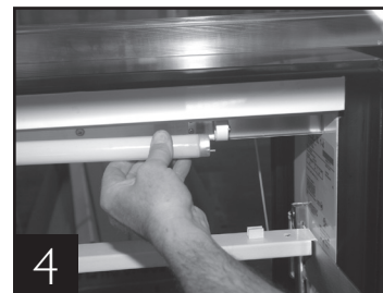
Remove bulb by gently pushing bulb into spring loaded lampholder.
