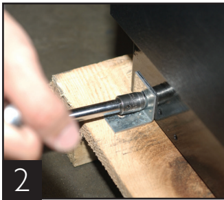
Removing bracket from cabinet.
