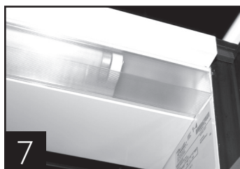
Interior top light assembly properly installed.
