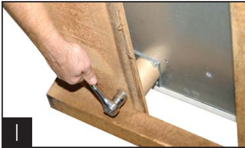
Removing skid from bottom of cabinet.
